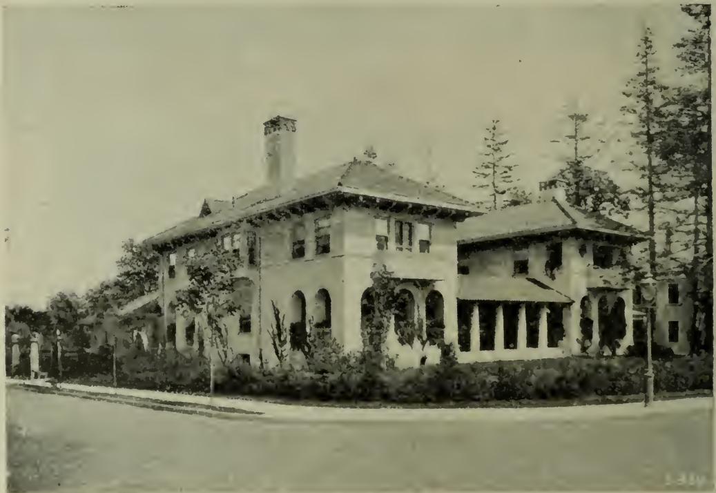
GENERAL VIEW—HOUSE AT FORT HAMILTON.
